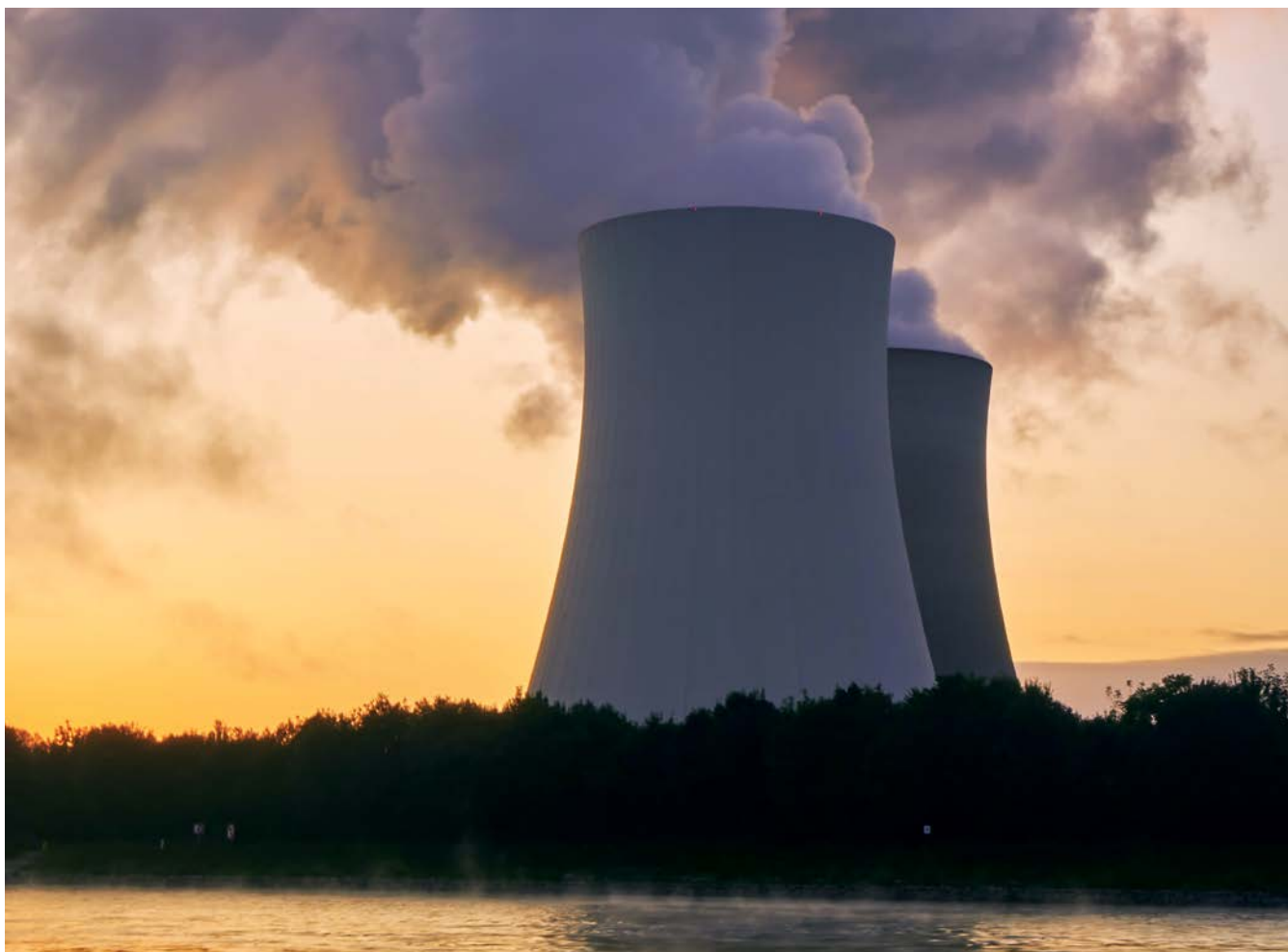
Photo: Coal Power Plants. (Image supplied by Markus Distelrath)
